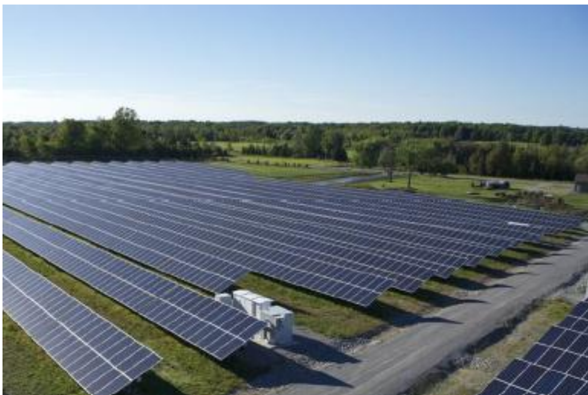
Image 4.2: Fixed South Facing PV Arrays
