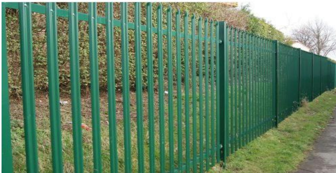
Image 4.14: Steel Palisade Fence
