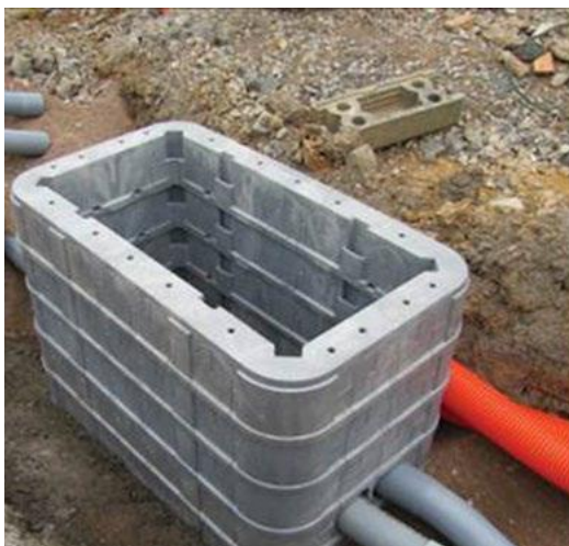
Image 4.12: Fibre Chambers (Construction and External Appearance)
