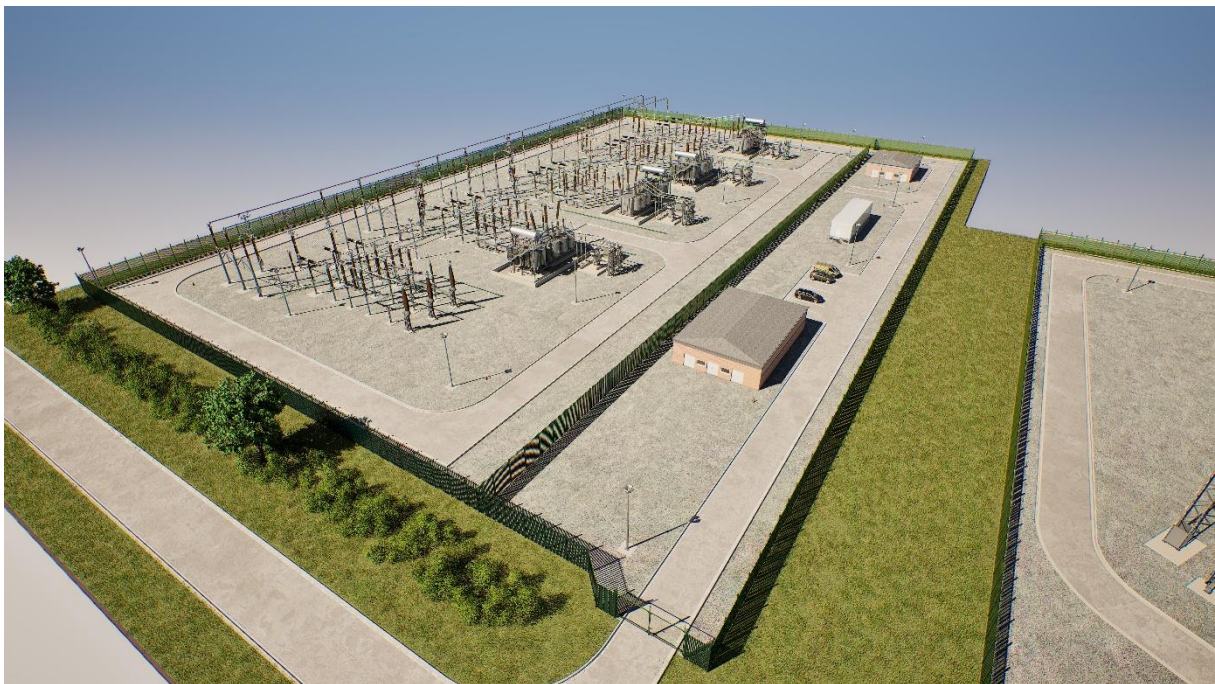
Image 4.10: Air Insulated Substation
