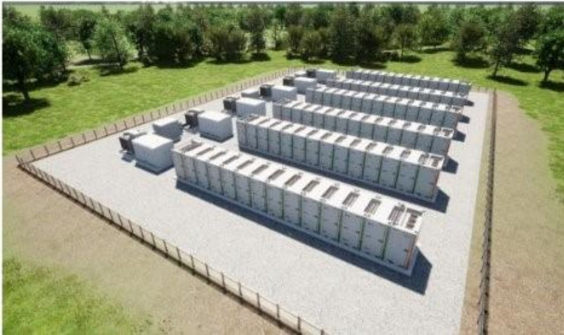
Image 4.7: Typical Battery and Energy Storage System
